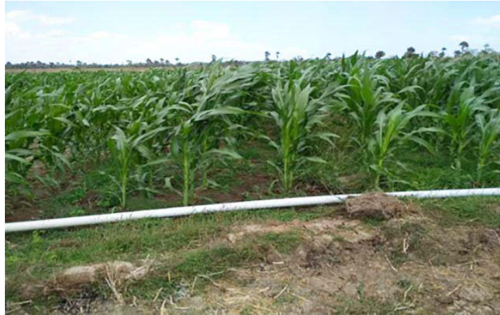
A PVC pipeline crossing a cornfield.
